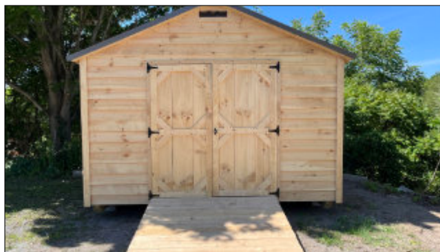
Figure 4: OVRRA's new shed
